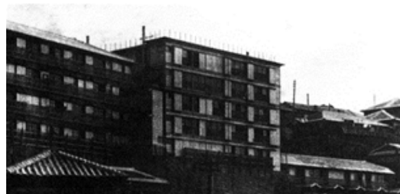
Fig.13 A five-story wooden building (Reinforced Concrete was used for the floors and roof), 1913
